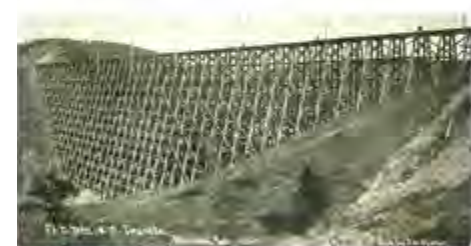
MODIFIED ON NEARBY BASS POINT CREEK TRESTLE BRIDGE FROM BOONE, IOWA
